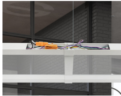
Slide fixture together and connect the connectors
